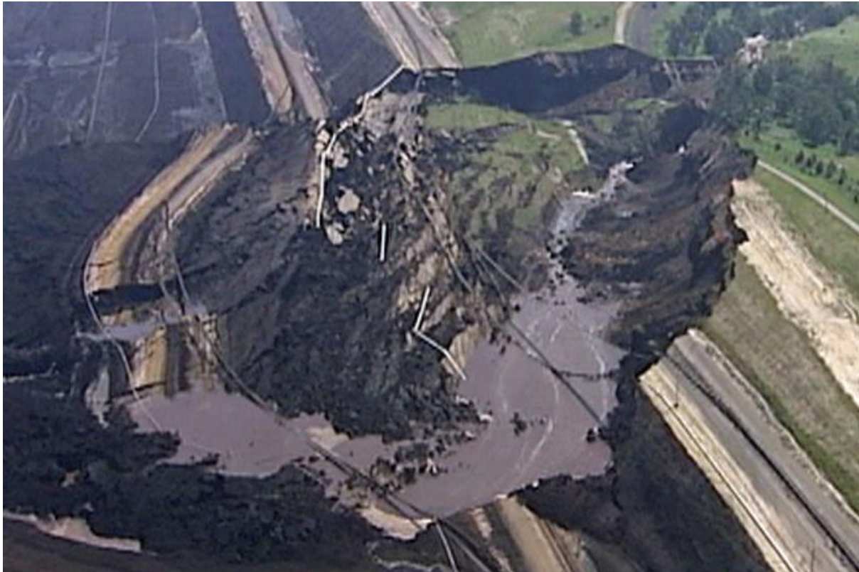
Aerial view of the damaged coal mine at the Yallourn Power Plant in eastern Victoria. (ABC-TV)
