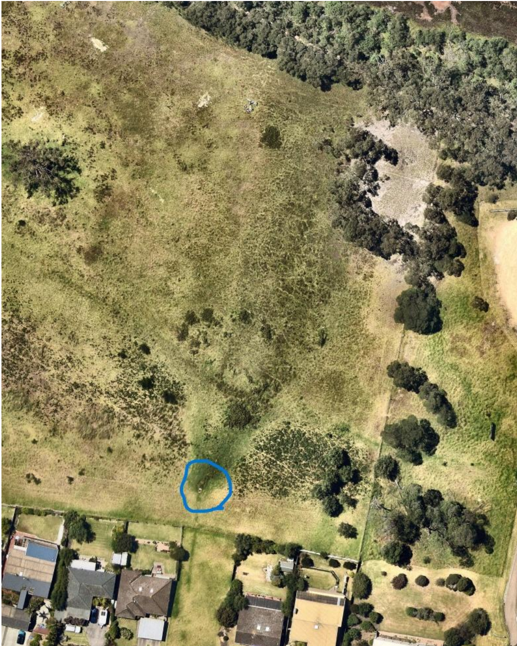
Figure 9: Nearnmap aerial view of the eastern outfall (circled in blue) - Photo taken Feb. 2024
